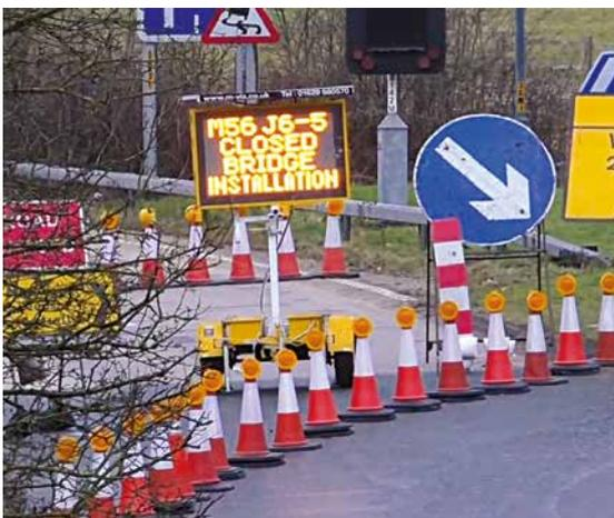
VMS were deployed at four closure points, with live streaming CCTV mounted on the same platforms. The VMS were surrounded by intelligent cone barriers and contactless sensors to detect breaches. VMS messages in advance of the workzone warned road users of the closure and surveillance.
